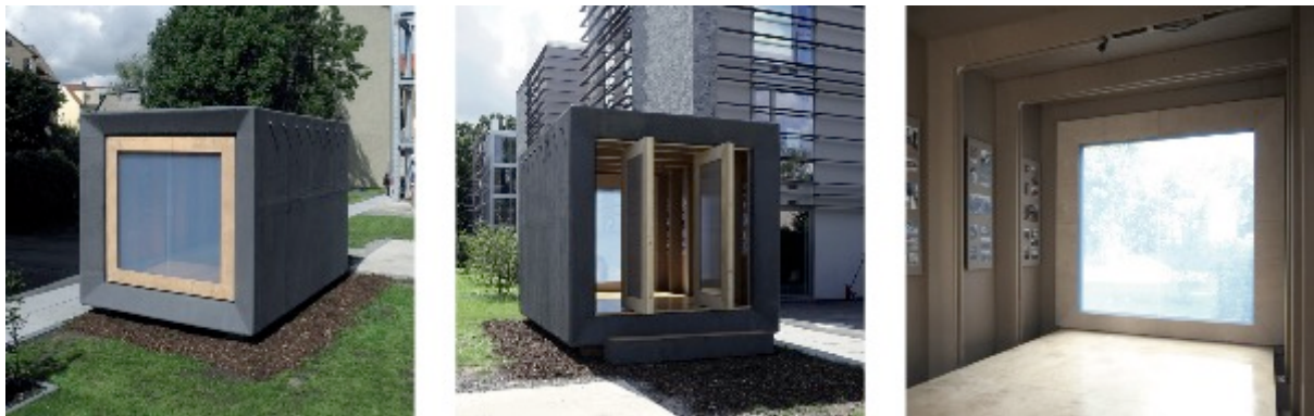
Figure 8: South facade (left), north facade (centre) and interior (right)
