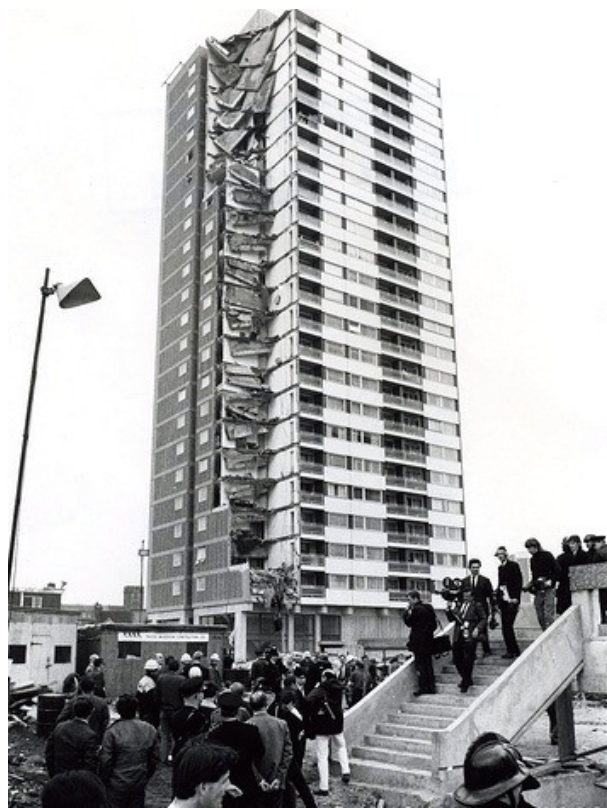
Figure 1: Progressive collapse of the Ronan Point Tower [7]
