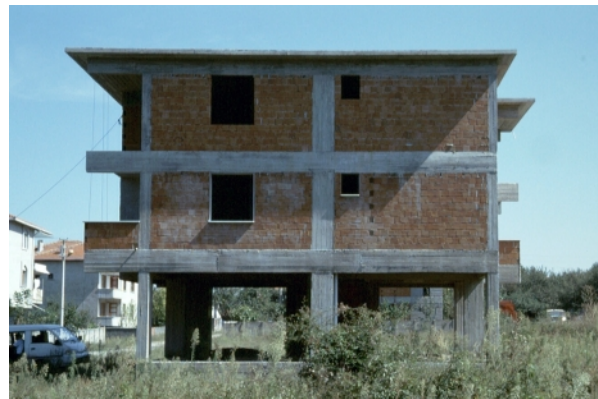
General view of the west facade
