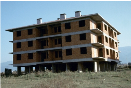
General view of the north facade
