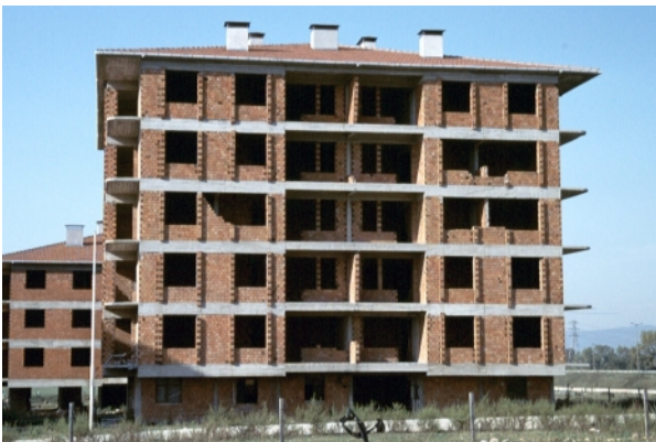
General view of the east facade
