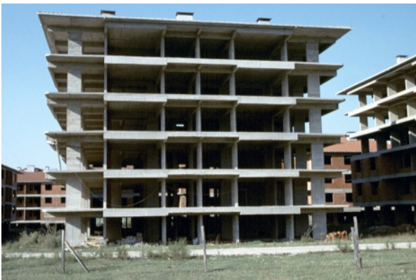
General view of the east facade
