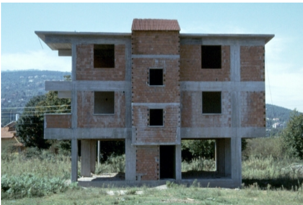
General view of the east facade
