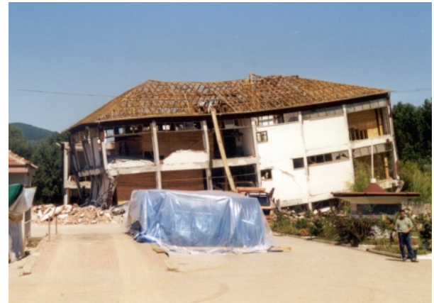
General view after the damaging 1999 İzmit (Kocaeli) earthquake
