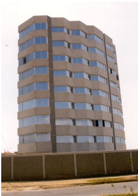
General view of the north facade
