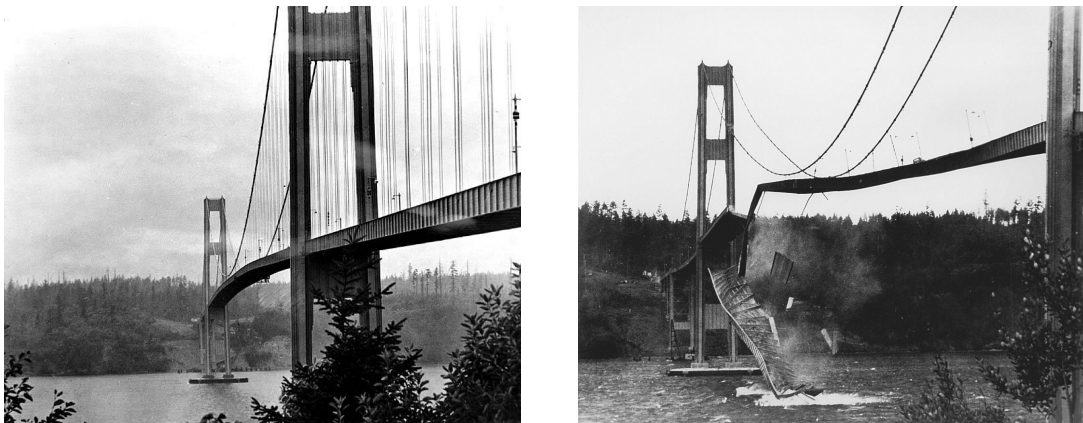
Figure 1.1: The Tacoma Narrows Bridge before (left) and after the collapse (right) (picture courtesy: University of Washington Libraries, Special Collections).
