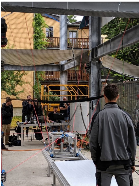
Fig. 10 Cable based 3D-printer mounted in an existing steel structure
