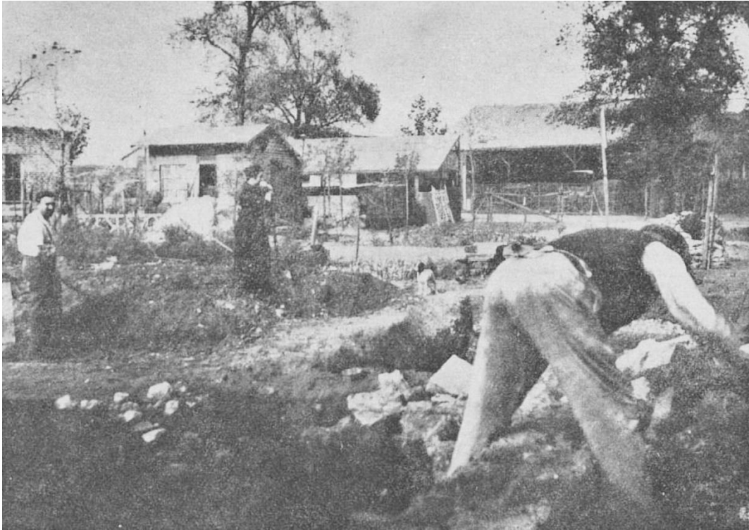
Photo 36. Bicoques under construction. Source: (Bisson, 1933, p. 363).
