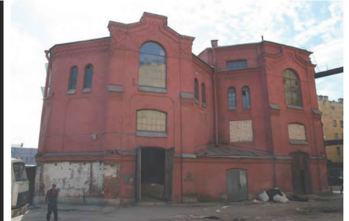
Andrey Vorontsov. "From the Historic warehouse of scenery for the Alexandrinka, two walls are remained - The News of Construction of St. Petersburg -Kanoner," Kanoner, September 19, 2010. Photo. Available from: http://kanoner.com/2010/09/19/17660/ . (accessed February 13, 2017). Copyright: Kanoner, Andrey Vorontsov. The use of image is granted by the owners.
