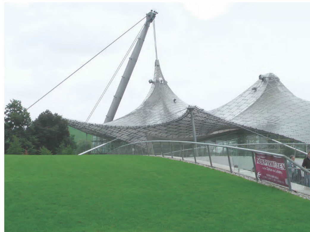
Olympia tent-roof construction. 1968-1972. Architect: Otto Frei.
