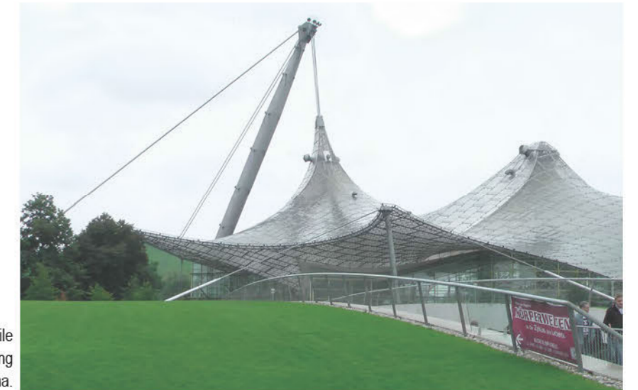
Swimming Arena The source of the image and construction description: Frei Otto and Ludwig Glaeser, The Work of Frei Otto (New York: Museum of Modern Art, distributed by New York Graphic Society, Greenwich, Conn, 1972), 112.
