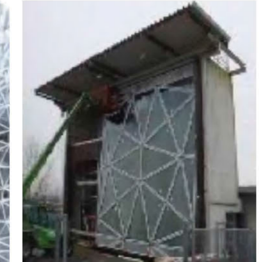
Screenshot from the conference video. Source: CTBUH. CTBUH 2009 Chicago Conference - Tony Kettle, "Gazprom Tower: The Politics of High Rise." 20:43. https://www.youtube.com/watch?v=M_C7FHzCJvM . (accessed 15 April, 2017)
