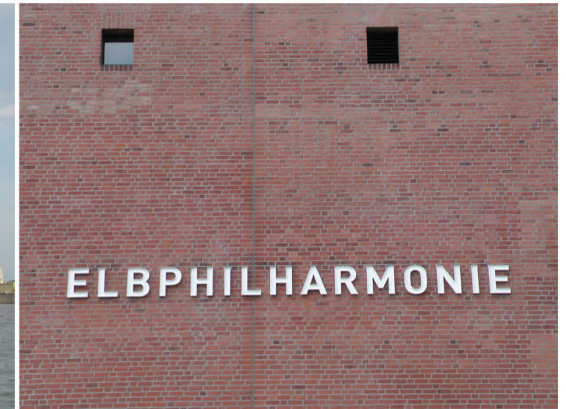
Reshetnikova T., 2016. The Elbphilharmonie brick facade.
