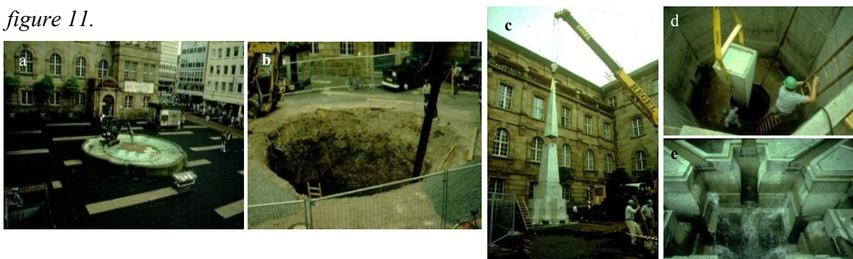
Figure 11: The fountain's construction as a reminder: a- Aschrottbrunnen Fountain Project. Removal of Original Base Used as a Flower Bed. b- Excavation for New Fountain Memorial c- Counter Monument Ready for Installation.d- Memorial Being Installed. e-Fountain Before Before Covered with Glass. Source: http://chgs.umn.edu/museum/memorials/hoheisel/fountain.html
