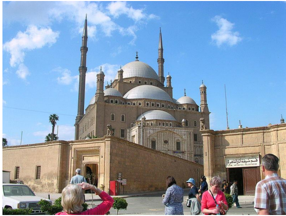
Figure 10: Muhammad Ali built his state mosque entirely in the Ottomans architectural style, the style of his former overlords. The Ottoman mosque has a central dome surrounded by four small and four semi-circular domes. It constructed in a square plan. Two elegant Turkish cylindrical minarets, two balconies, and conical caps are on the western side of the mosque which rises to 82 meters. The external facades are severe, angular and rise about four stories until the level of the lead-covered domes. Source: https://ar.m.wikipedia.org/wiki/%D9%85%D9%84%D9%81:M.Ali_Mosque2.JPG
