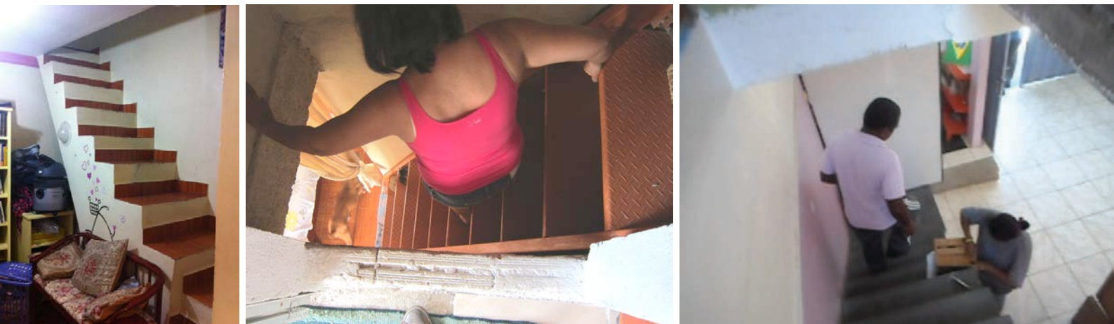
Stairways from Flavia, Carlota and Eduardo. People can hit their heads on the beams. Author's file, 2013.
