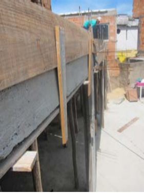
Wooden formworks. Author's file, 2013.
