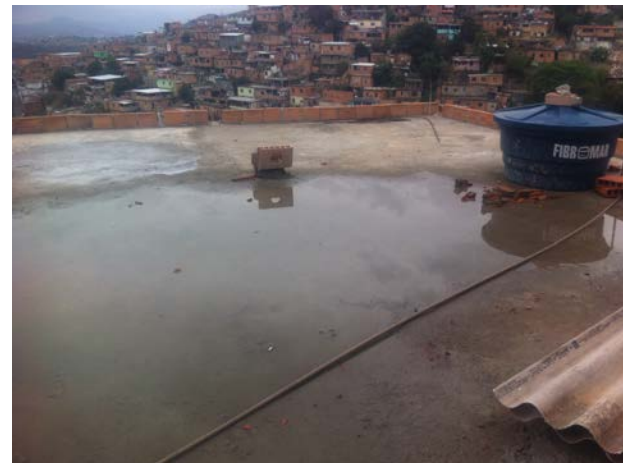
Uncovered concrete slab waiting for the next floor. Author's file, 2013.
