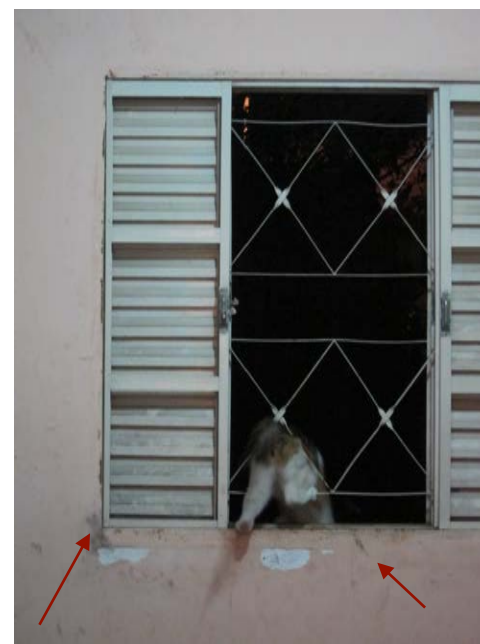
Window without lintel and sill. The red arrow indicates infiltrations spots. Author's file, 2013.
