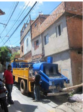
Concrete pumping machine. Author's file, 2013.
