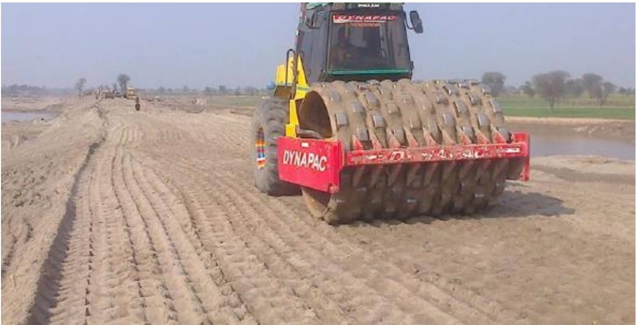
Figure 5-1: Compaction of formation bed
