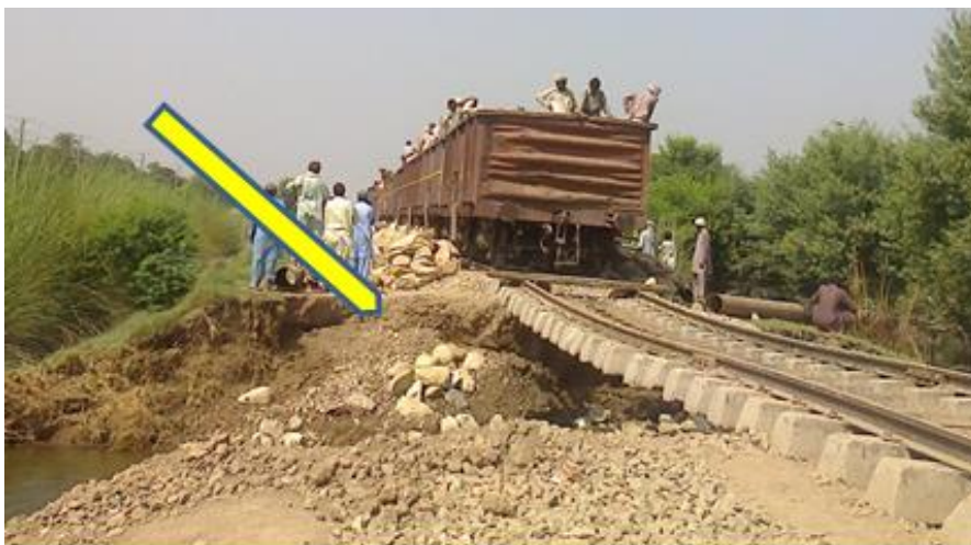
Figure 1-2: Embankment failure
