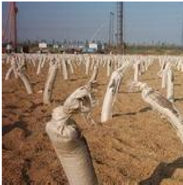
Figure 5-2: Working on packed drains in progress
