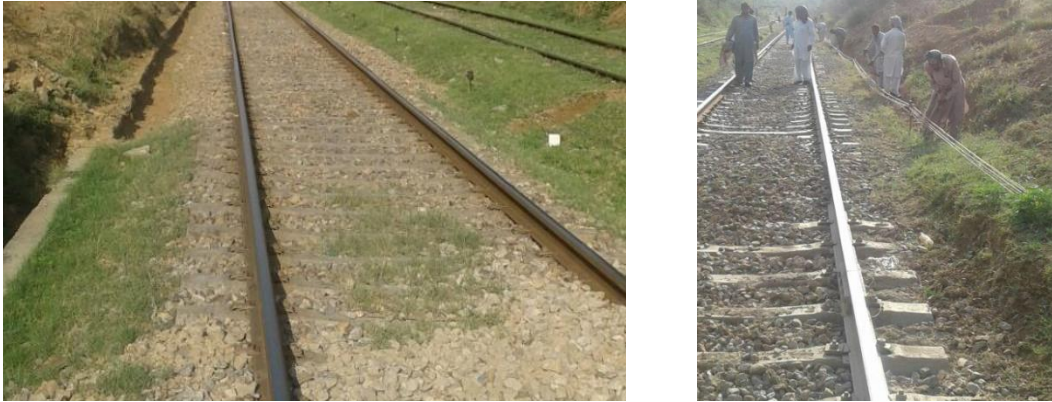
Figure 7-4: Kacha & pacca side drains
