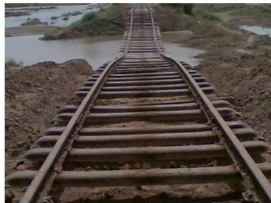
Figure 1-3: Overflow of flood water and side drains
