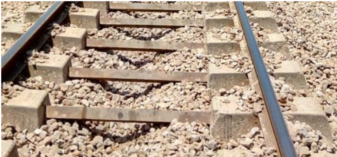
Figure 7-1: Twin block sleepers in Main line (Rawalpindi to Lahore section)
