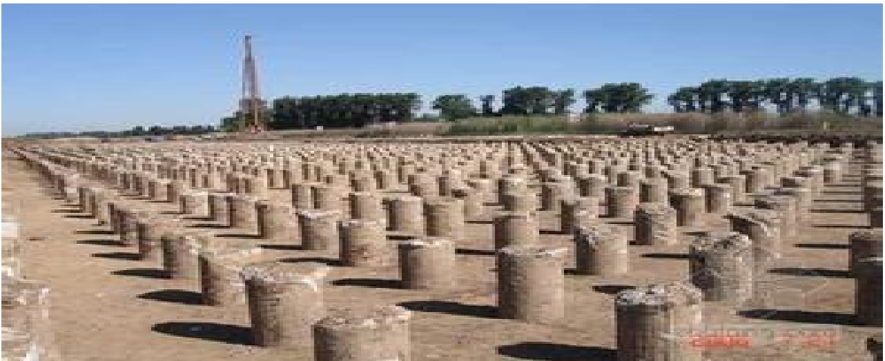
Figure 5-5: Piles in yard
