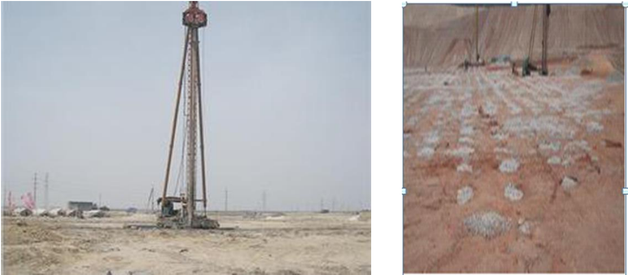
Figure 5-4: Stone column installation process
