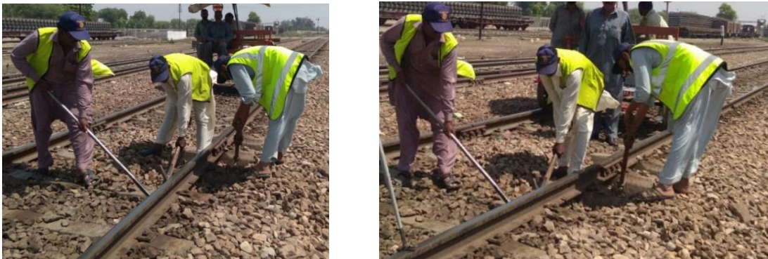
Figure 7-3: Track maintenance through labors (manually)
