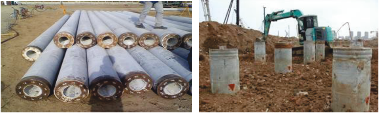
Figure 5-6: Pre-stress piles
