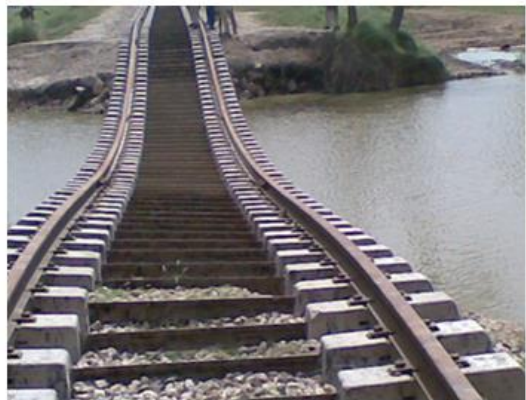
Figure 1-3: Overflow of flood water and side drains
