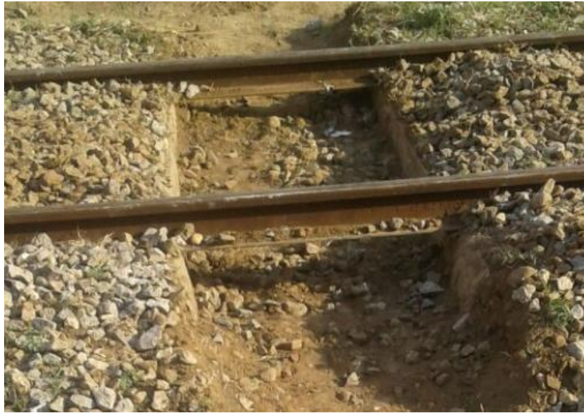
Figure 6-4: Ballast mixed with soil layer
