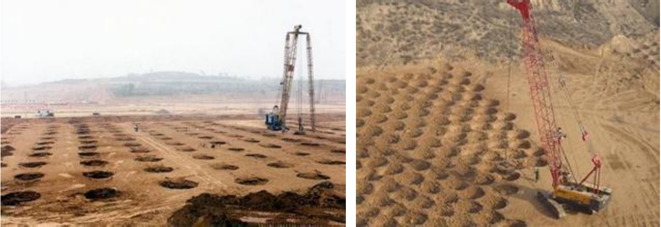
Figure 5-3: working on dynamic compaction in progress
