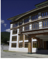
6 - office building with brick infill walls
