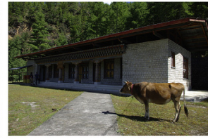
5 - local government building constructed with natural stone in cement mortar
