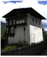
1 - rammed earth with timber-frame rabsel
