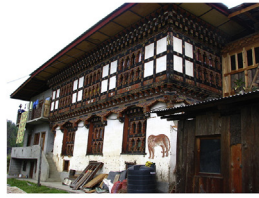
2 - contemporary rammed earth house with timber-frame rabsel
