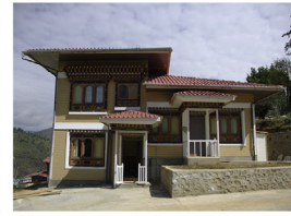
4 - contemporary house with 3 flats built with cement stabilised earth blocks
