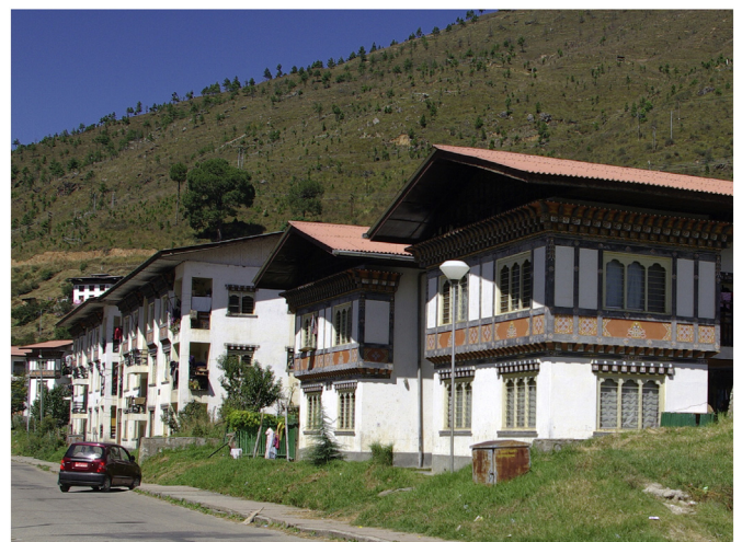
Fig. 2. Government constructed apartment buildings in Thimphu in reinforced concrete frame construction with brick infills and concrete formwork for architectural design elements.
