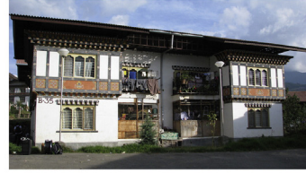
8 - social housing with multiple flats in reinforced concrete frame construction with brick infill walls
