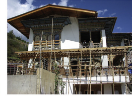
10 - reinforced concrete frame house with aerated concrete blocks
