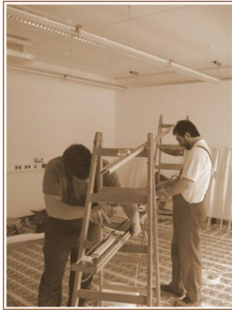
Electrical workers block entirely a room for their work
