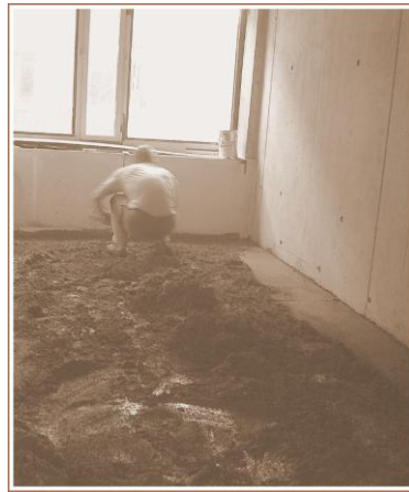
A worker must block a whole room for screeds
