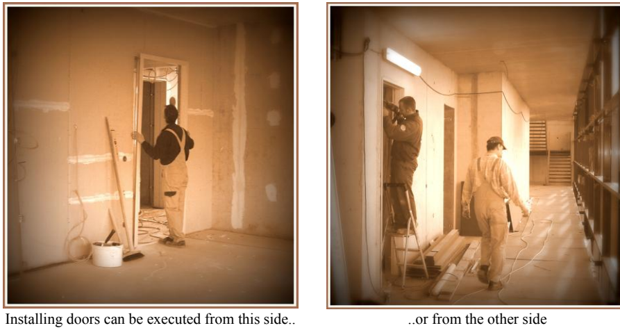
Figure 2.11: Possibilities of workspace allocation for installing doors
