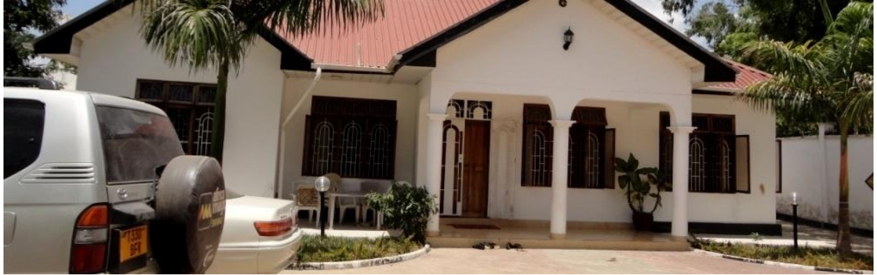
Figure 39: Bugler proof materials on windows and doors
