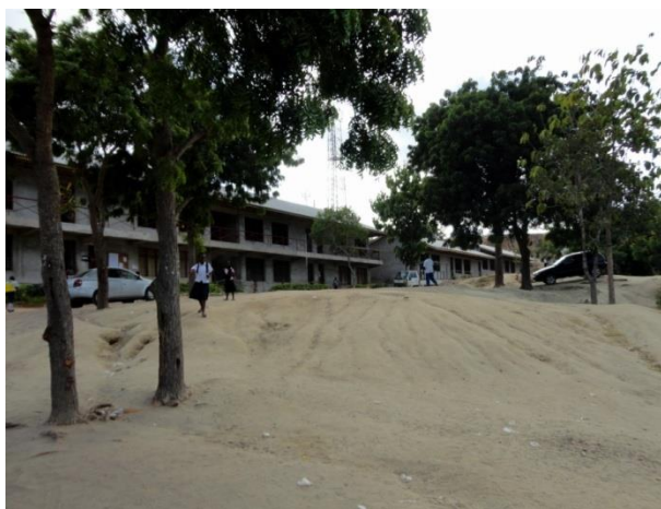
Figure 113: Ronda primary and secondary school
