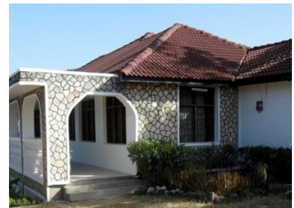
Figure 34: Plastered concrete blocks, stone cladding walls and tiled roof
