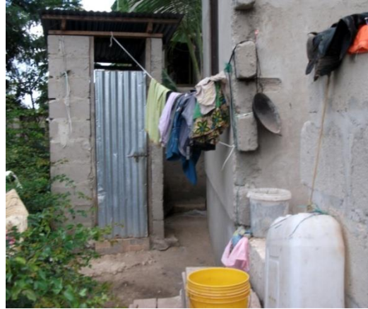
Figure 78: An outdoor dry pit latrine
