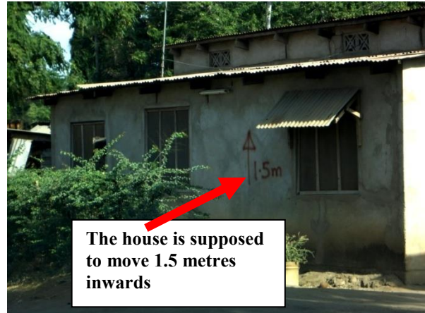
Figure 102: A house demolition mark to allow road expansion
