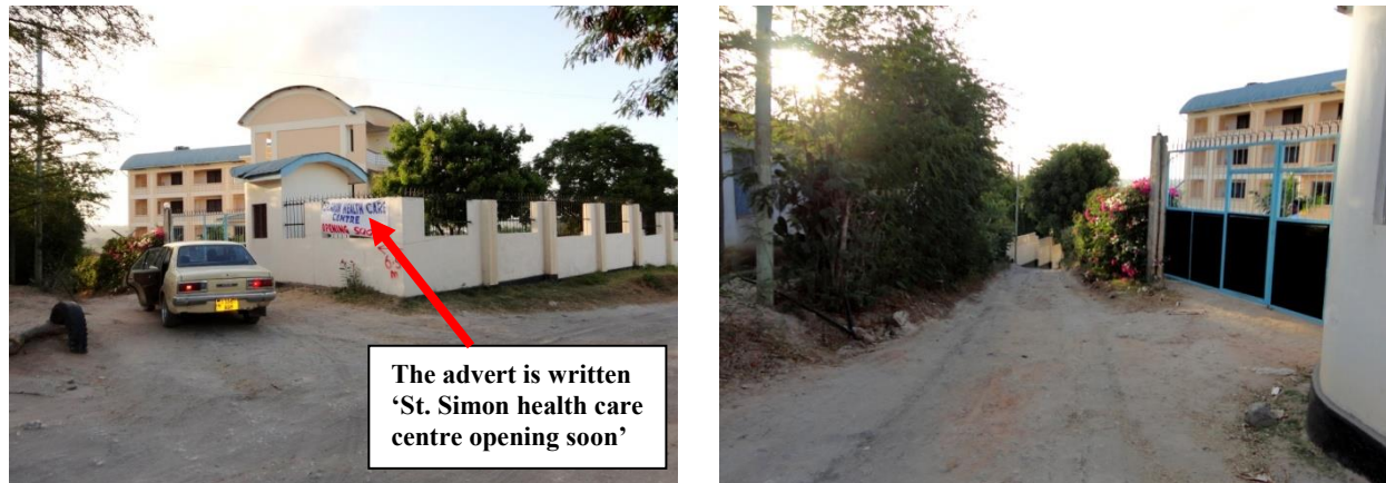
Figure 117: A private hostel building to be changed into a health centre
