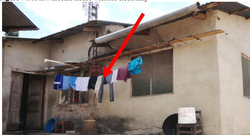
Figure 75: A middle income house with electricity
