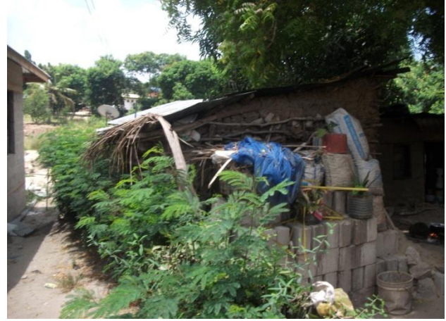
Figure 47: Concrete blocks piled for further construction
