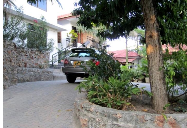
Figure 82: A sloppy site and costly site works
