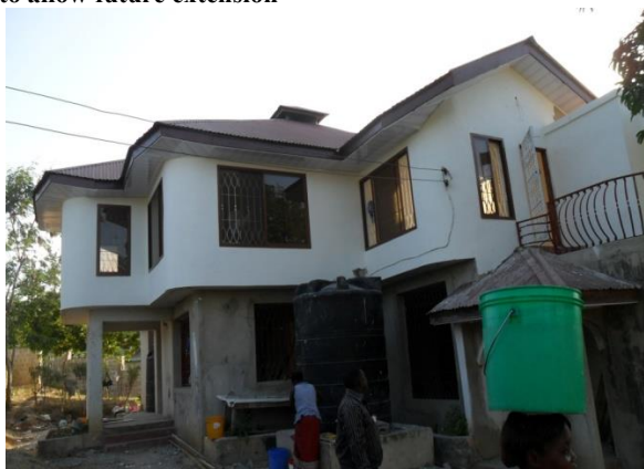
Figure 50: Incremental building by a high income
