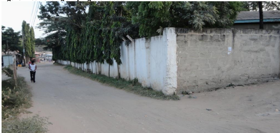
Figure 121: A sharp corner created by a fence in the foreground
