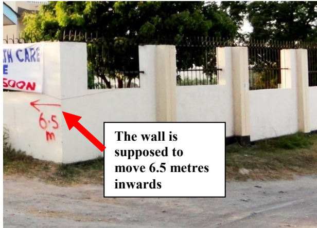
Figure 101: A fence demolition mark to allow road expansion
