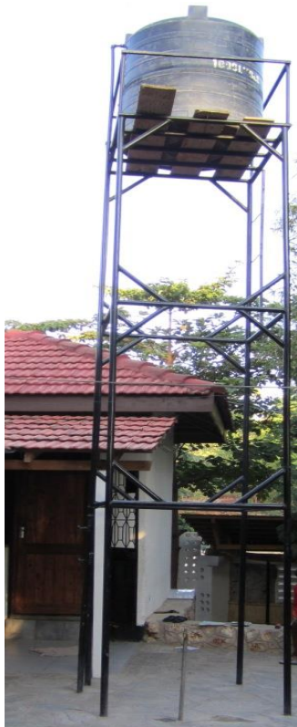
Figure 66: Water is pumped up from a bigger tank
