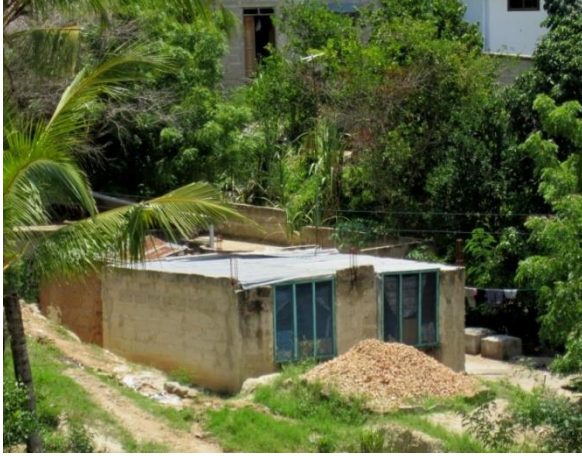
Figure 46: Gravel piled for further construction
