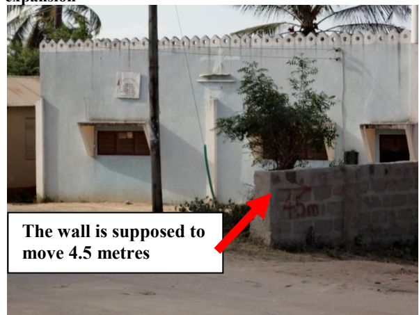
Figure 104: A half wall along Makongo road marked to be demolished
