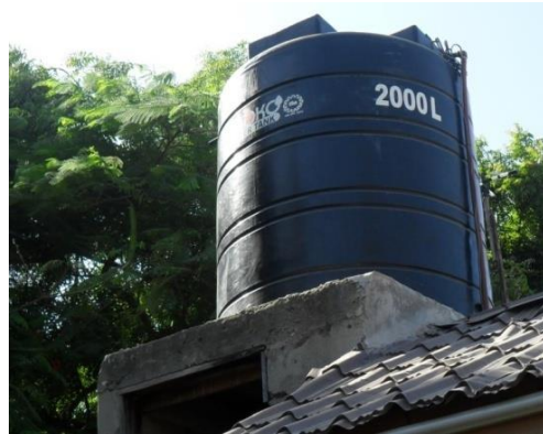
Figure 67: Water is pumped up and flow by gravity
