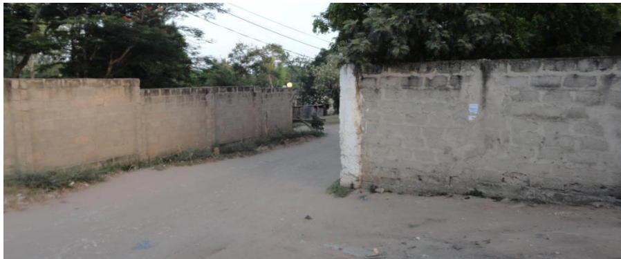
Figure 120: Fencing shaping the road
