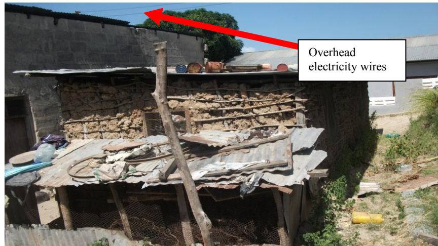
Figure 74: A low income house without electricity
