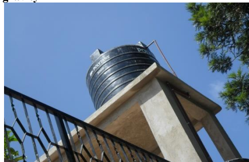
Figure 69: A 3000 litre simtanks on a concrete structure
