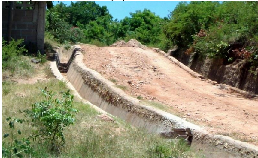
Figure 99: Privately constructed drainage channels along the private road
