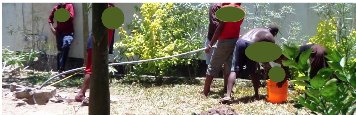
Figure 96: Digging 100 metres underground (borehole) to get water
