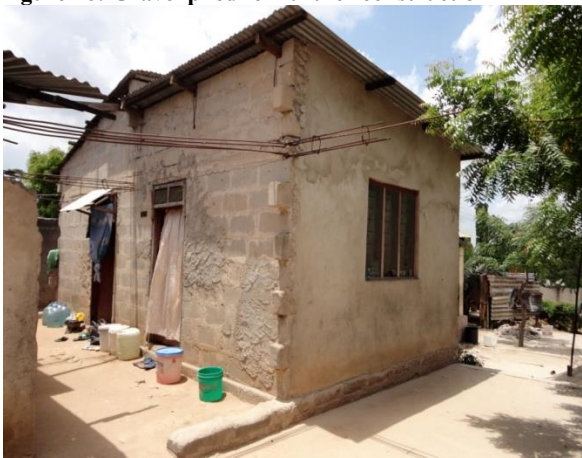
Figure 48: Extended foundation and reinforcement bars to allow future extension
