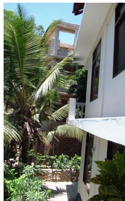
Figure 58: Another apartment building under construction at the far end
