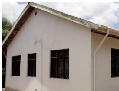
Figure 33: Plastered concrete blocks and corrugated iron sheets roof
