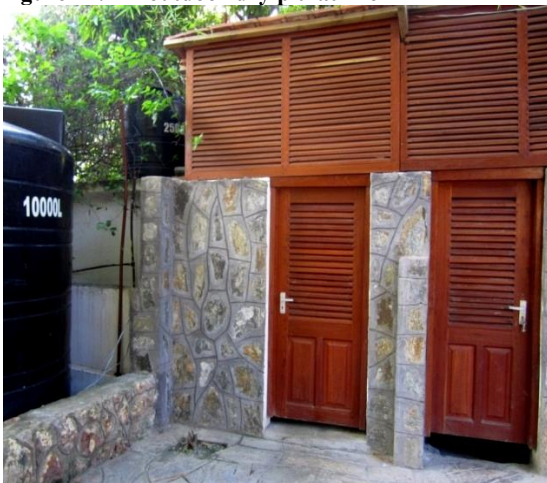
Figure 79: A toilet in a high income house compound
