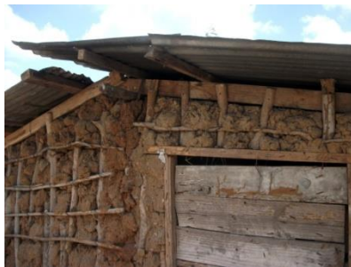
Figure 32: Corrugated iron sheets roof
