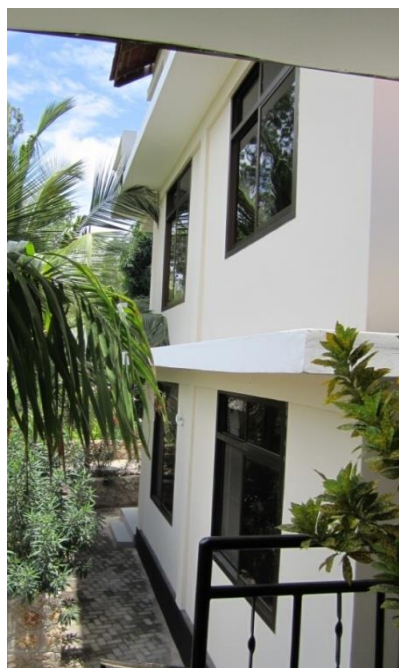
Figure 57: Front view of the apartment building extension
