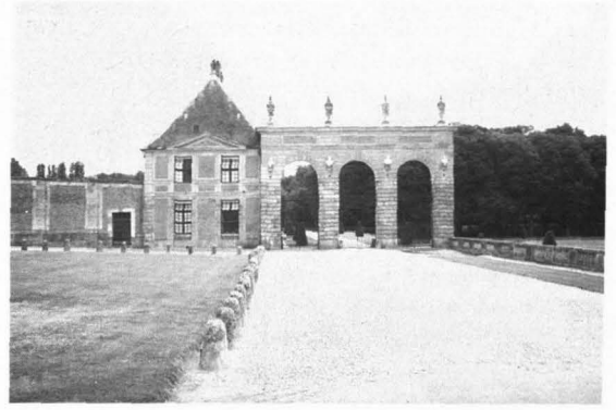
G View of wing-wall
